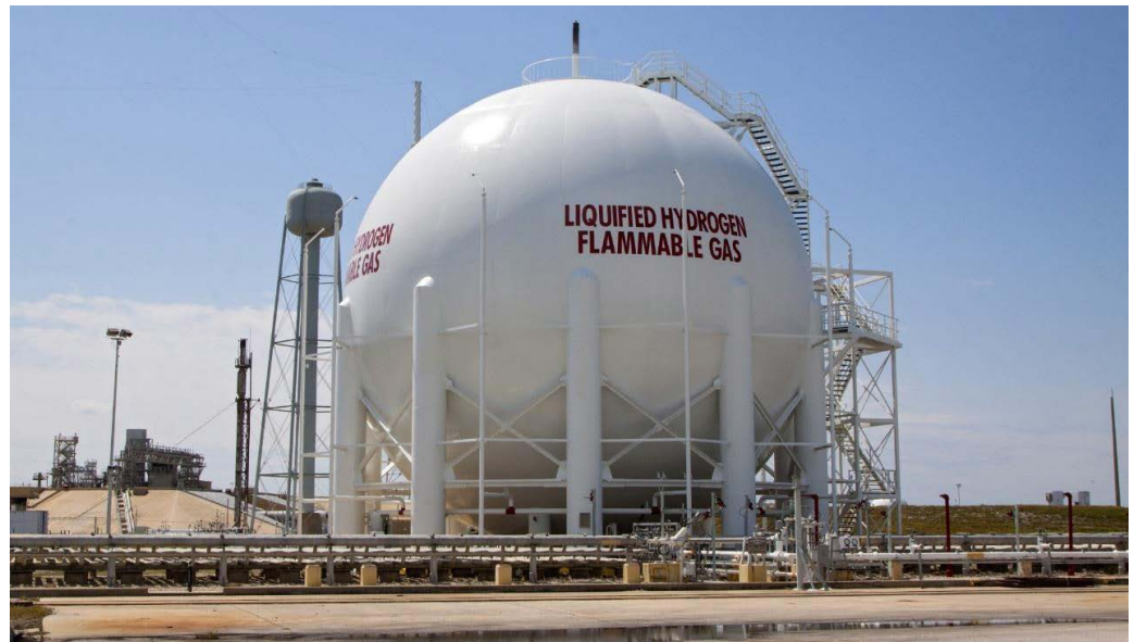
Figure 24 Liquefied hydrogen storage, 3200 m 3 in the Kennedy Space Centre, USA
