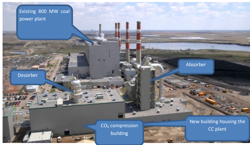
Figure 13. Photo [37] of Saskpower 800 MW e Boundary Dam coal-fired power station where one of the four units was retrofitted with amine CC in 2013.
