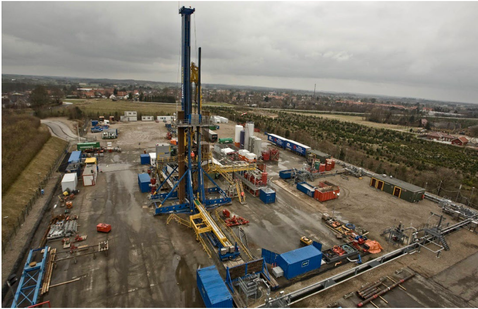
Figure 0-32: Drilling operation at injection well pad [9]
