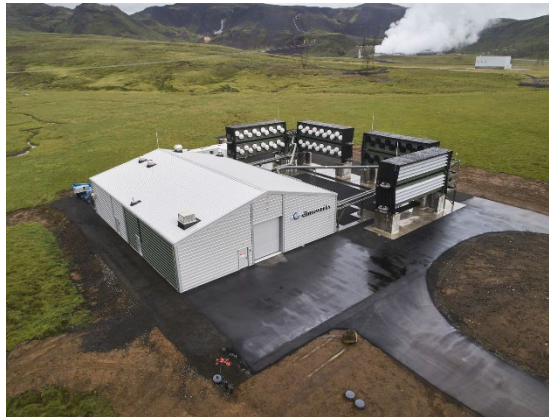
Figure 42. Climeworks largest direct air capture plant located in Iceland [3].
