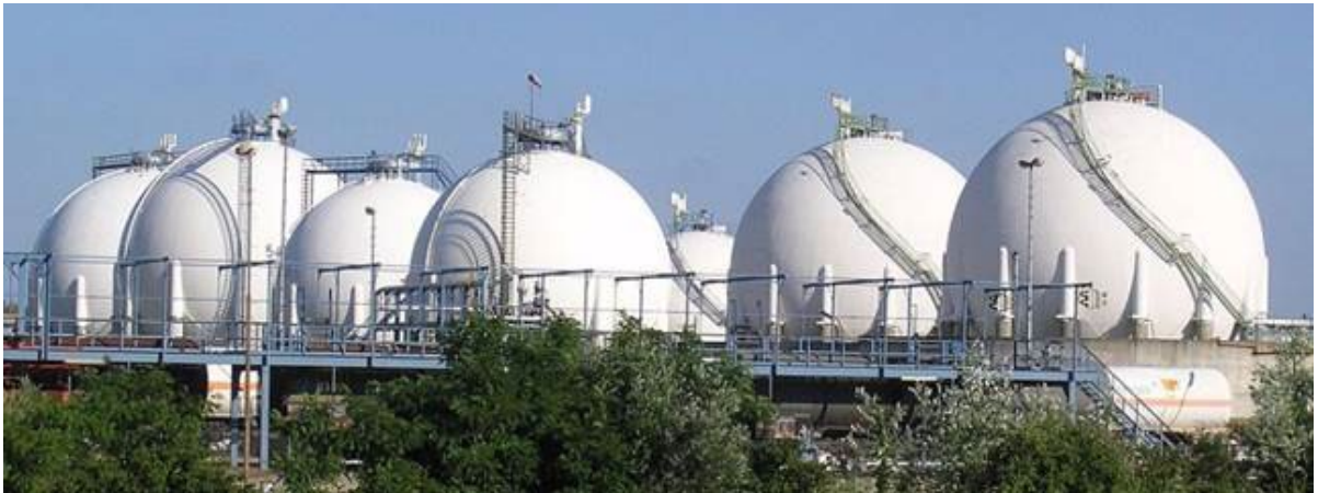
Figure 0-29: Typical gas storage tanks [21]
