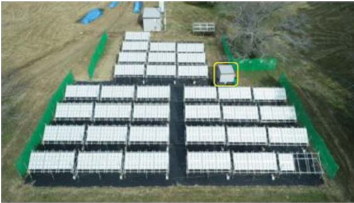
Figure 12.8 An overhead view of the 100-m 2 photocatalytic solar hydrogen plant based on NCCs installed at Kakioka Research Center (Japan). Source: Nishiyama et al. [70]/with permission of Springer Nature.
