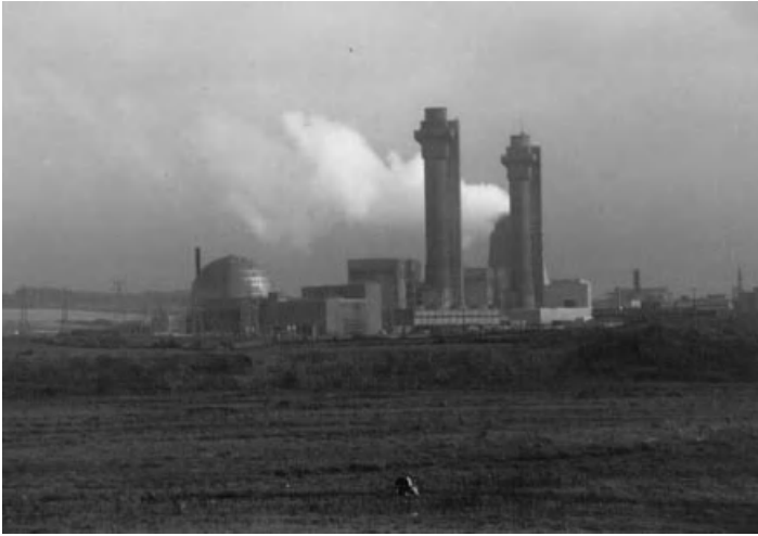
Figure 60 Photograph of the Windscale Piles being decommissioned (Chris Eaton, October 2009). Source: http://www.geograph.org.uk/photo/330062 .
