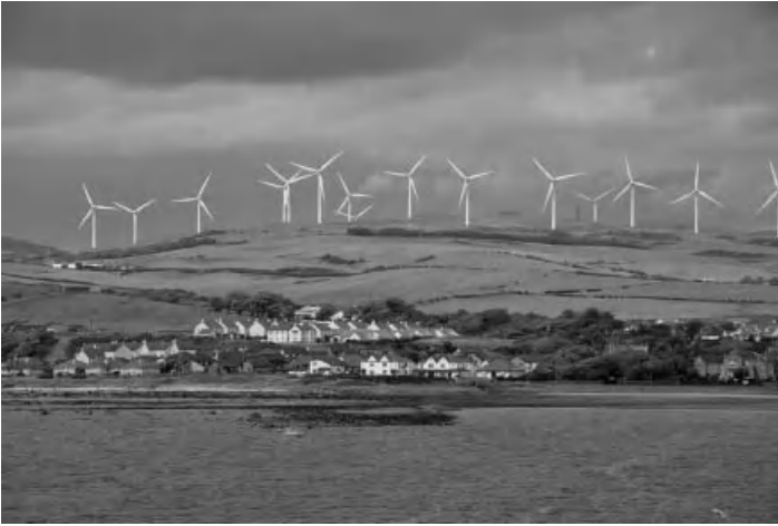
Figure 62 Skyline of the Ardrossan wind farm, North Ayrshire, Scotland. Note the houses in front. Photo by Vincent van Zeijst, July 3, 2010. Source http://en.wikipedia.org/wiki/File:Ardrossan,_Scotland,_United_Kingdom.JPG .
