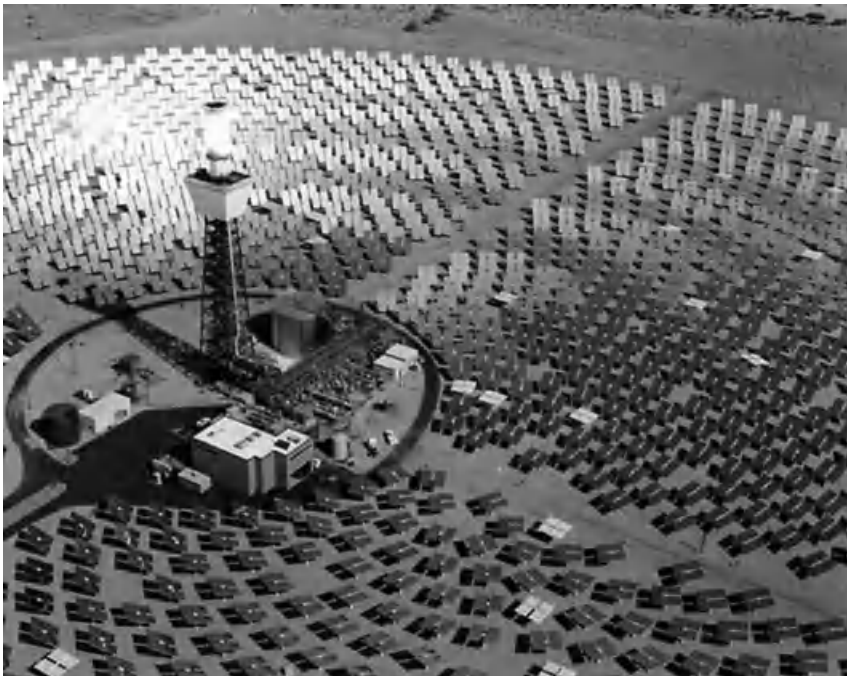
Figure 52 Aerial view of the Solar Two facility, showing the power tower (left) surrounded by the sun-tracking mirrors. Source, http://earthobservatory.nasa.gov/Features/RenewableEnergy/Images/solar_two.jpg .
