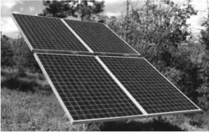
Figure 19 Solar panels that convert sunlight into electricity. Photo: Tom Grundy/Shutterstock.
