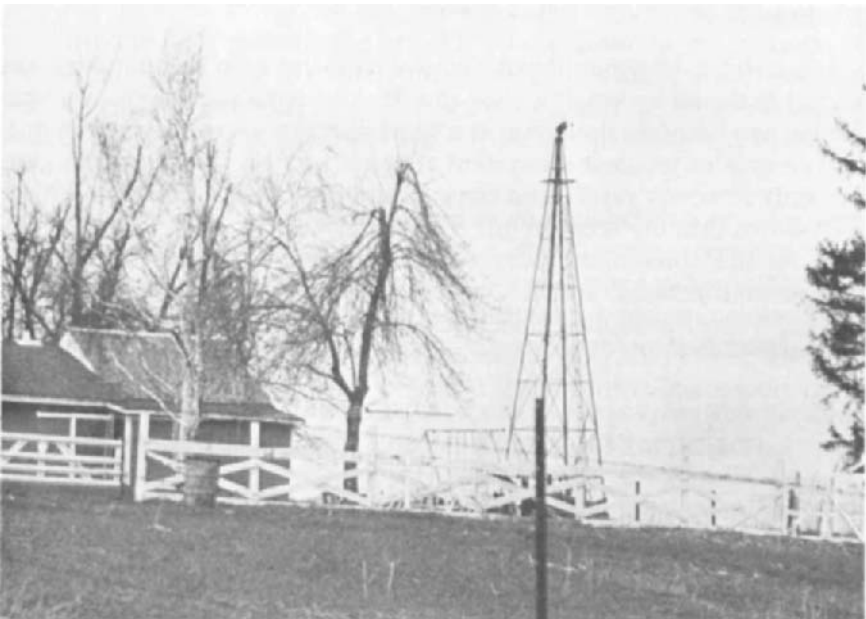
Fig. XIX.1. Ice-storm destruction 13 months earlier is still evident in trees near Mineral Point in southwestern Wisconsin.
