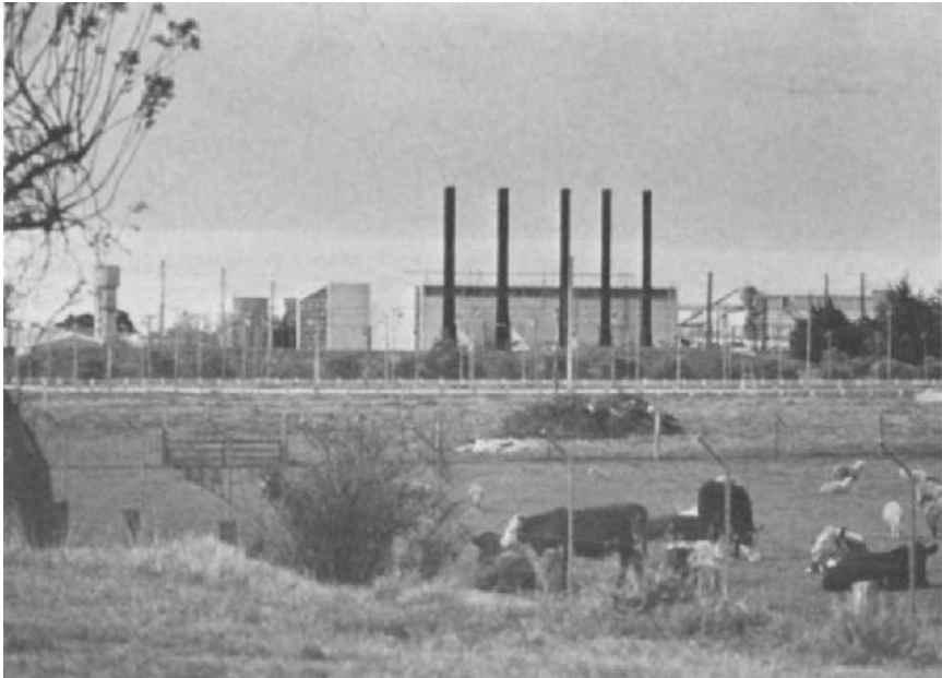
Fig. XXII.1. Electricity-generating plant at Mt. Gambier, South Australia, burns residues from logging and milling of plantation pines that are more or less contemporaneous biological energy.
