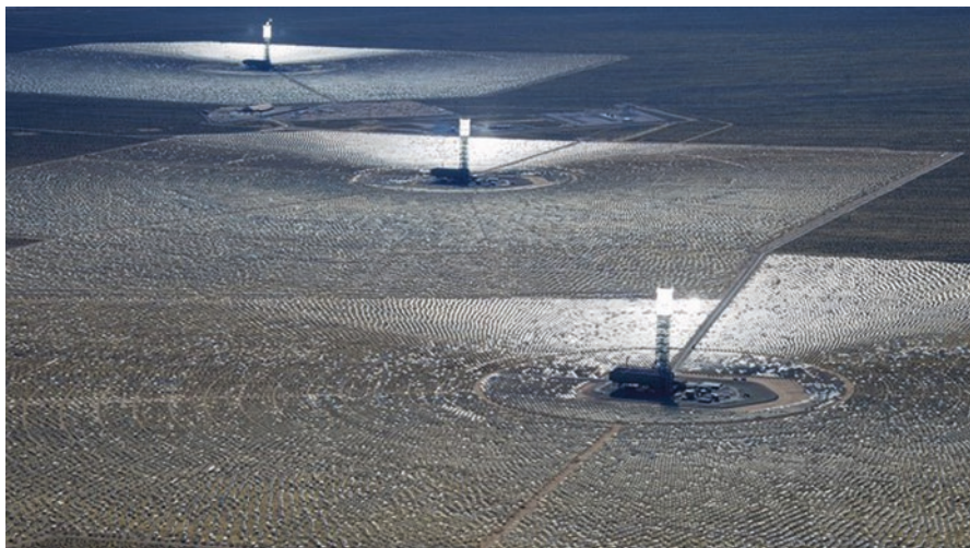
Fig. 7.3 The solar thermal power plant located on Ivanpah Dry Lake in the Mojave Desert of California. Arrays of mirrors focus sunlight onto the central towers, creating heat. The plant has a peak output of 392 MW. (Source: U.S. Department of Energy photograph; public domain)
