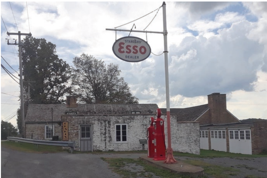
Fig. 3.5 Depression-era Esso service station from 1934 preserved in the “New Deal” town of Arthurdale, West Virginia. (Source: Photographed in 2021 by Dan Soeder)
