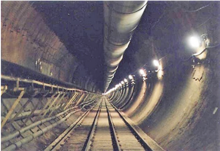
Fig. 7.8 The north ramp of the five-mile-long exploratory tunnel under Yucca Mountain in Nevada. (Source: Photographed in 1997 by Dan Soeder)
