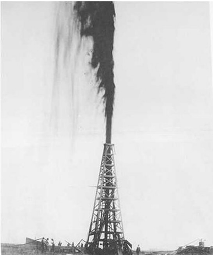
Fig. 3.3 The oil gusher from the Lucas well in January 1901 at Spindletop Hill, Texas. (Source: Wikimedia Commons public domain; original photo by John Trost)
