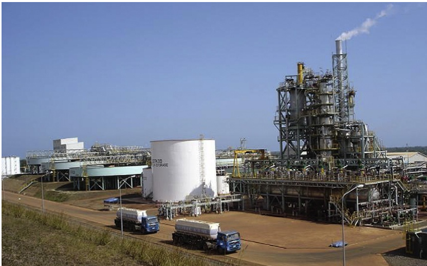
FIGURE 11.1 High-temperature sulfide leach plant at Coral Bay, Philippines. It processes the limonite layer of the laterite deposit and produces a mixed precipitate of nickel and cobalt sulfides, which is shipped to Niihama, Japan for refining to high-purity nickel and cobalt. The autoclave is on the lower right, sulfuric acid storage tank is in the center and the thickeners are on the left. The flash-tank tower is above the autoclave. Source: Photograph courtesy of Sumitomo Metal Mining Ltd.
