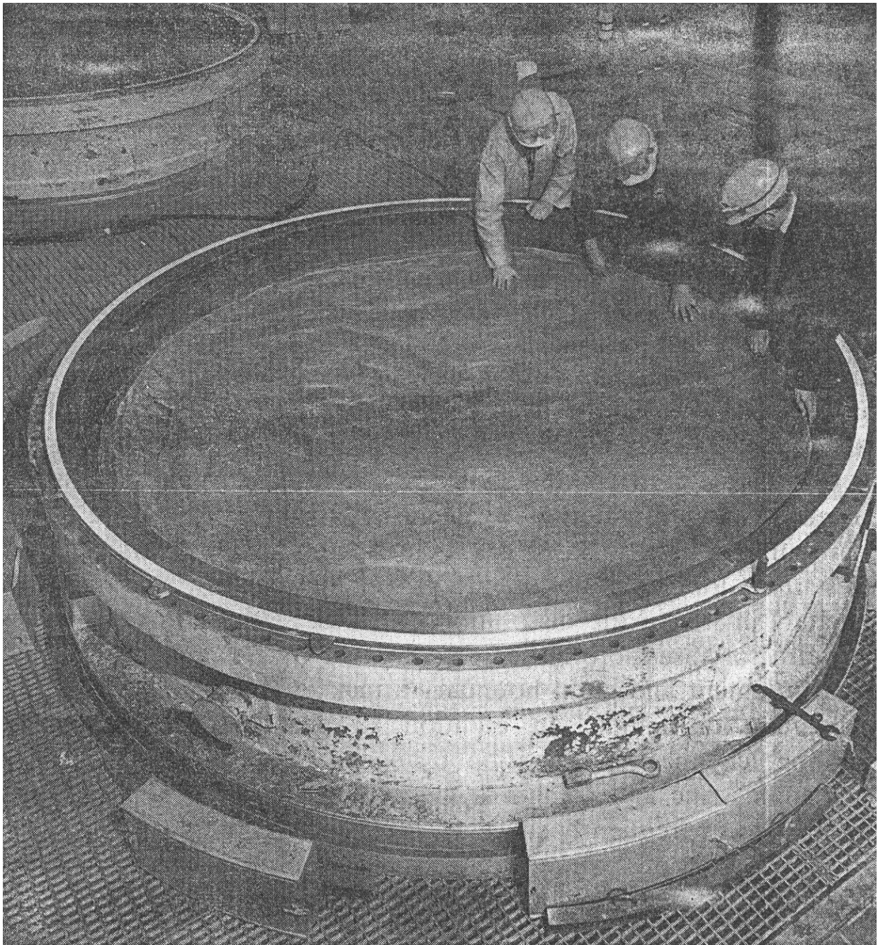
Figure 10.12. Installation of gauze pad—checking for wrinkles.
