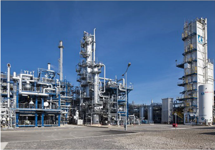
Fig. 3.2 Industrial steam methane reformer. Source Air Liquide; see: https://www.airliquide.com/media/air-liquide-starts-large-hydrogen-production-unit-germany
