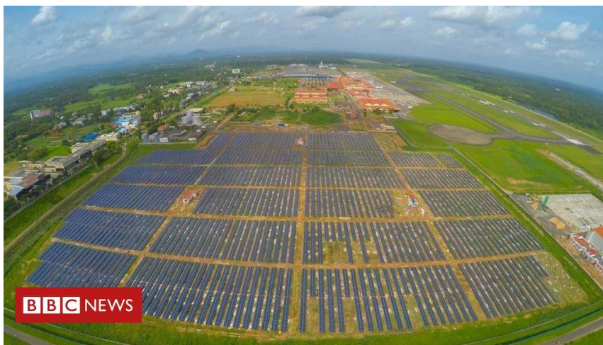
Figure 1 Solar power plant at Kochi airport producing 12 MWp; 46,150 solar panels laid across 45 acres
