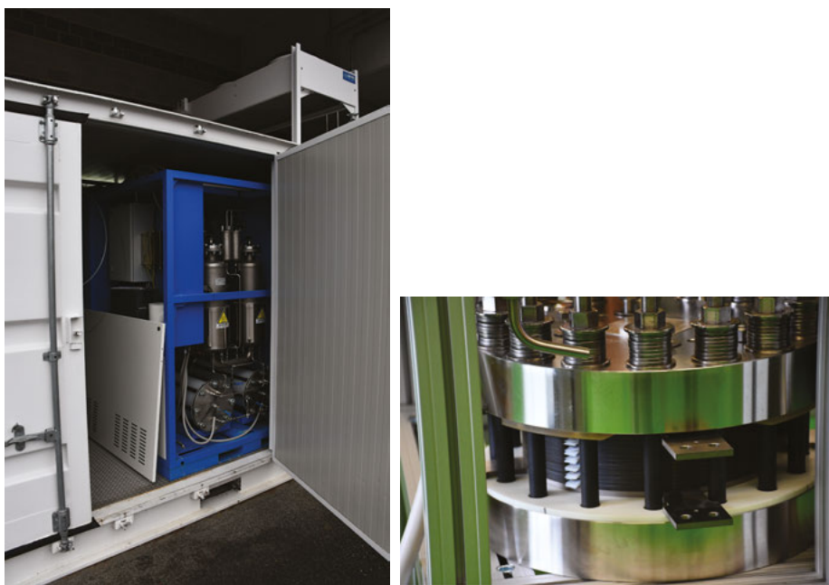
Figure 3.6: Custom-built alkaline electrolyzer system with two stacks (50 kW, 10 bar, “long”), and a custom built PEM electrolyzer (25 kW, 40 bar, “short”) at the hydrogen filling station in Martigny, Switzerland [Ligen 2018].
