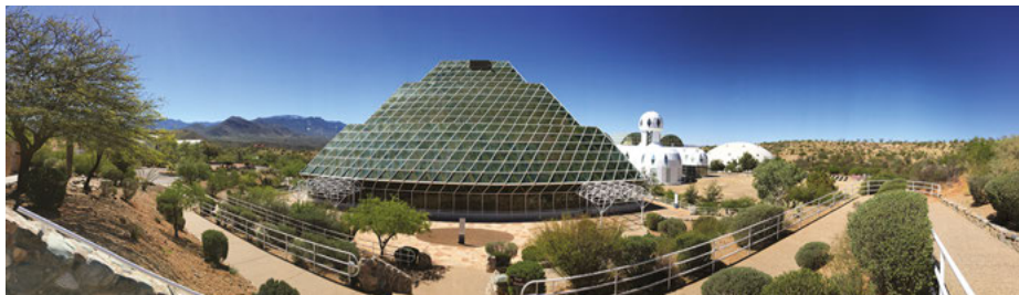
Figure 11.13: Biosphere 2 building complex in Oracle, Arizona. The large hermetically closed greenhouse with glass windows hosts a tropical rainforest, savannah and desert climate regions in addition to a large water basin. The white buildings are connected and served as working and living areas for eight humans. The half-dome is the energy supply center.
