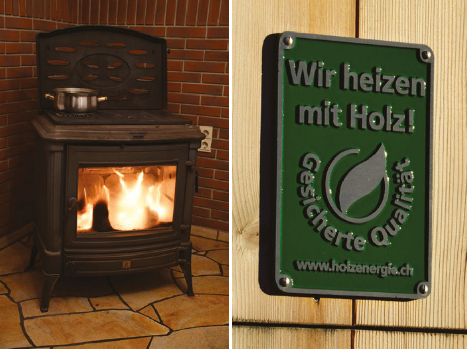
Figure 9.8: (left) An iron stove in a residential home. Wooden logs are burnt in the stove and release the heat in the room. The flow of air into the stove can be optimized so that only minimum soot is produced. A pipe at the backside of the stove leads smoke and carbon dioxide through the wall to the rooftop of the home into the environment. The ash from the burnt wood is collected in a tray at the bottom of the stove and can be emptied regularly. New wood logs are fed to the stove by opening the front door. With proper adjustment of the air flow in the stove, the logs can burn for several hours and provide a homogeneous flow of heat in the room. (right) We are heating with wood! Secured quality.” A slogan from the Swiss wood energy association, posted at a home in a remote rural area where wood is a major supply of energy for the residential homes.
