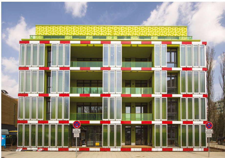
Figure 12.21: Arup, Strategic Science Consult (SSC) and Splitterwerk Architects, BIQ House, Hamburg, 2013. This first algae-powered building is covered with over 100 bio-reactive panels. Reproduced with permission from Wiley, Kolarevic B: Actualising (Overlooked) Material Capacities. Architectural Design 2015, 85:128–133, and Joannes Arlt, and laif. [Kolarevic 2015].
