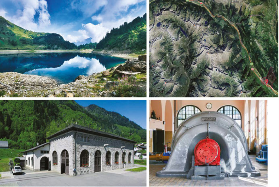
Figure 4.12: (top left) Lago Tremorgio which delivers water to Azienda Elettrica Ticinese, the mountain lake power plant building which houses the electric generators (lower left). (top right) Map showing Alp mountains, position of Lake Tremorgio and City of Bodio. (lower right) Electricity generator from Brown Boveri. Photos from Azienda Elettrica Ticinese, CH-6513 Monte Carasso.
