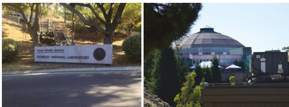
Figure 10.22: (Left) Access road (Cyclotron Rd.) to Lawrence Berkeley National Laboratory (LBNL) in Berkeley, California. (Right) The dome of the Advanced Light Source at LBNL. The structure is still from the 1930 when Ernest Orlando Lawrence built the large cyclotron.
