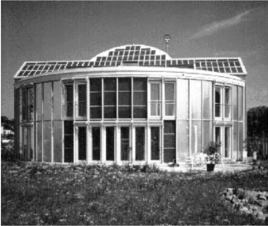
Fig. 57: Self-Sufficient Solar House in Freiburg, Germany utilizing hydrogen technology
