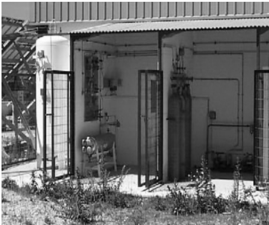
Fig. 53: Storage System: intermediate buffer (left), horizontal hydride container tank (middle), and 200-bar bottle and compressor (right).
