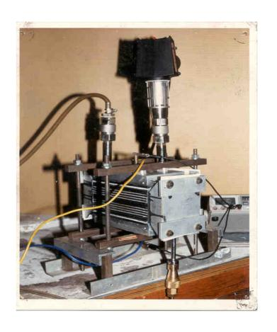
India's first kW rated Fuel Cell Stack (PAFC, 120x360 mm, 40 Cells, 1 kW) (1991)
